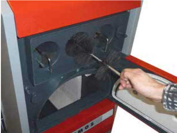
Cleaning of (tubes) exchanger with inserted the brush (by boiler D20P, D30P, D40P, D50P)
